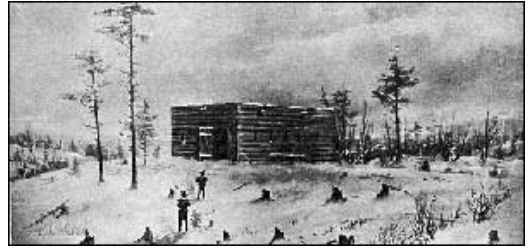
Building the Common House
